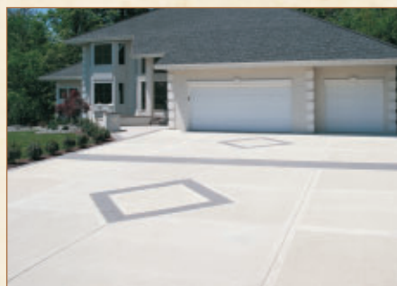
Concrete Driveways and Sidewalks
