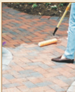
Apply by roller or spray
